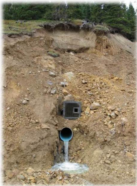
Gold King Level 7 Old Portal Closure
