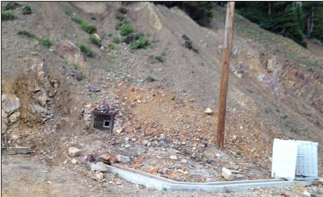
Figure 22.—Photograph showing the condition of the Gold King Level 7 New Adit portal on August 27, 2014, prior to any EPA modifications. Soil and rock debris have migrated downslope and covered a portion of the drain installed in 2009 (photograph from EPA project files).
