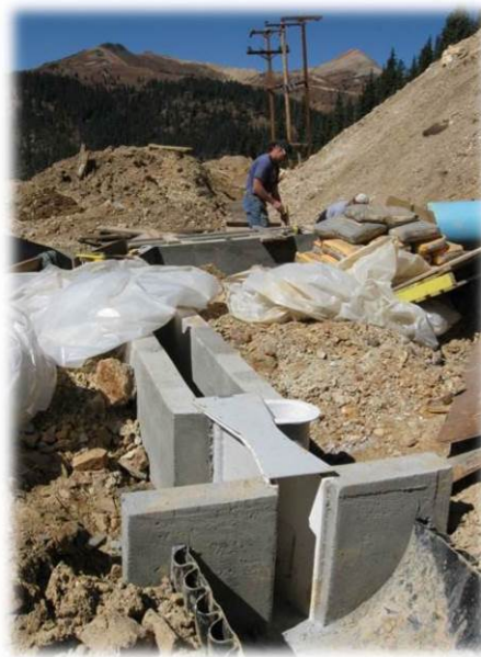
Gold King Level 7 Old Portal with 2" Parshall Flume Installed in Concrete Lined Ditch
