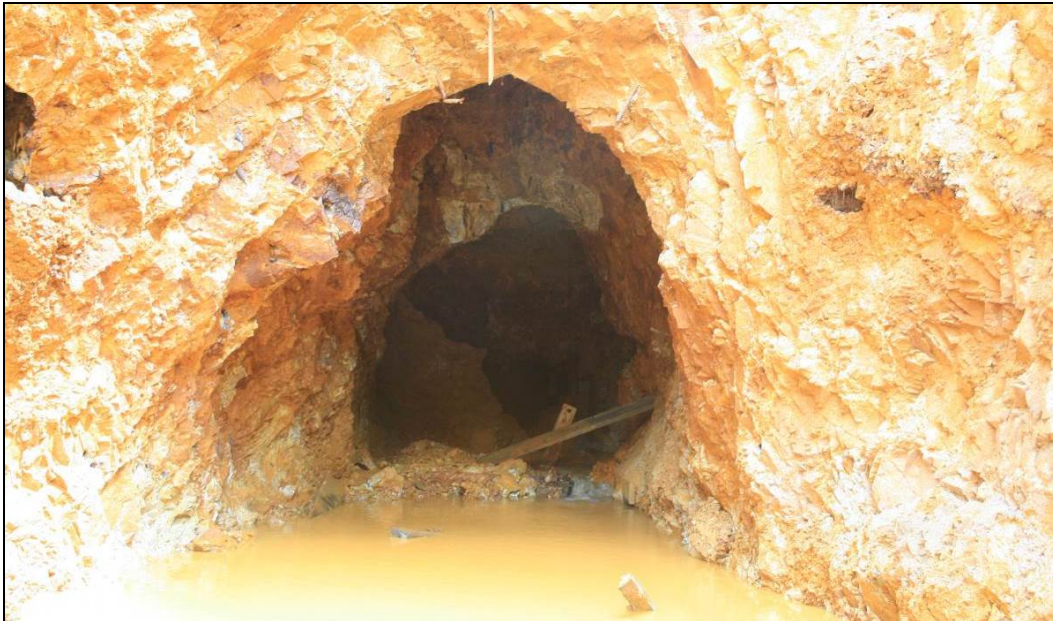
Figure 62.—Photograph showing the Gold King Mine Level 7 New Adit on August 16, 2015, after an excavator was used to reach inside the mine opening and remove the timbers. Note piles of debris from partial roof collapses inside the adit.
