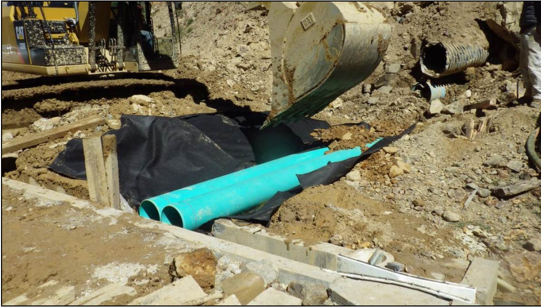
Figure 28.—Photograph taken on September 11, 2014, showing the installation of two new 2-foot-diameter drainage pipes. An entrance slot has been cut into the concrete trough for the pipes to discharge into (photograph from EPA project files).
