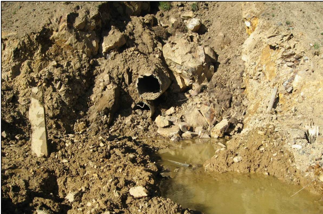
Figure 26.—Photograph showing the excavation of the Gold King Mine New Adit portal on September 11, 2014, taken shortly after the photograph in figure 23 (photograph from EPA project files).
