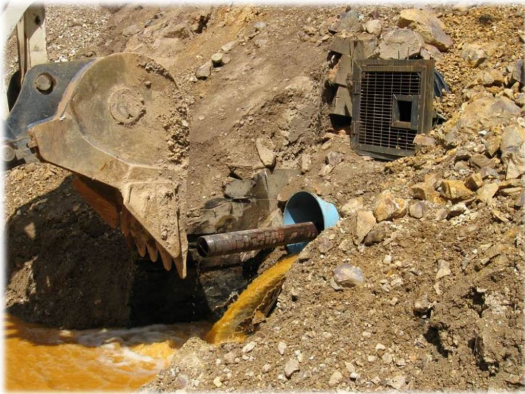
Gold King Level 7 Old Portal with well-point installed through the drain pipe. This portal may be re-opened in a future project to help stabilize the mine drainage and prevent future increases in mine pool head.
