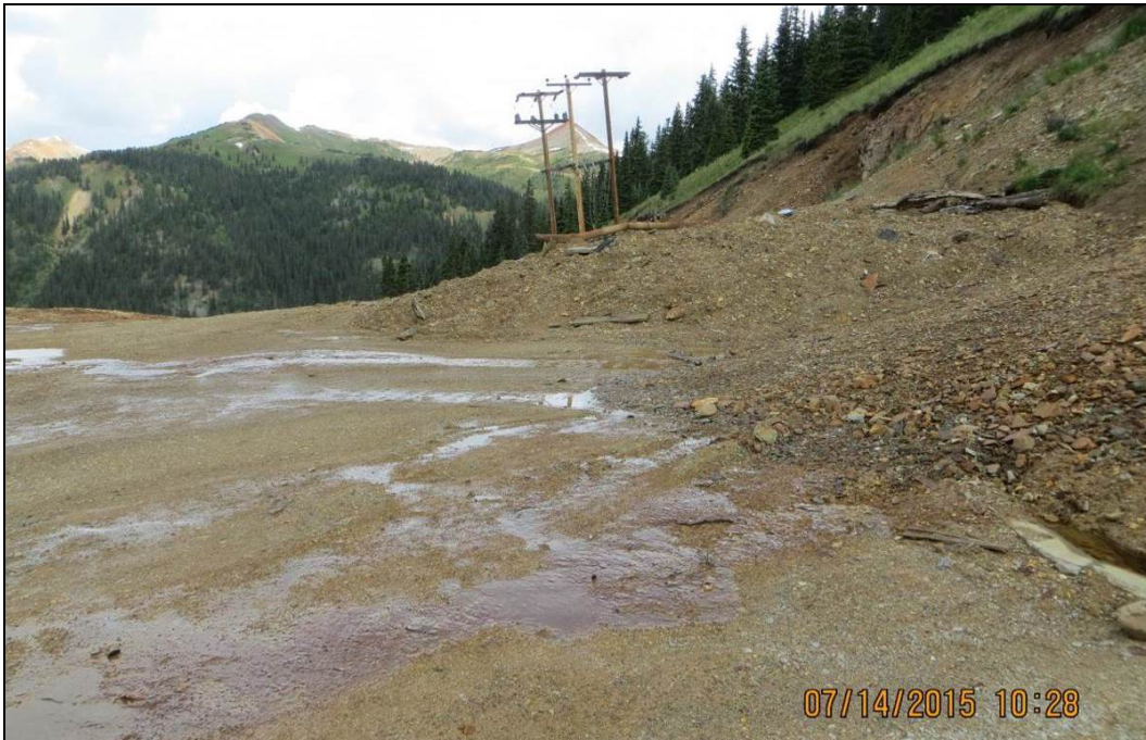
Figure 33.—Photograph showing the condition of the Gold King Mine Level 7 Old Adit portal area on July 14, 2015. Note that more soil and rock had slid from the slope area and had buried a portion of the concrete diversion channel including the ends of the two drain pipes (photograph from EPA project files).
