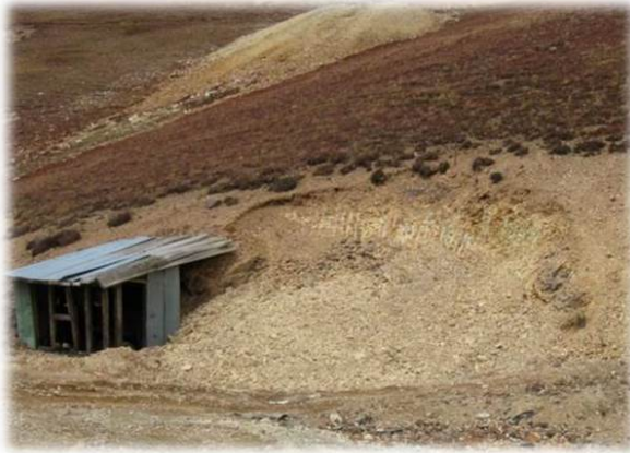
Number 1 Portal backfilled
