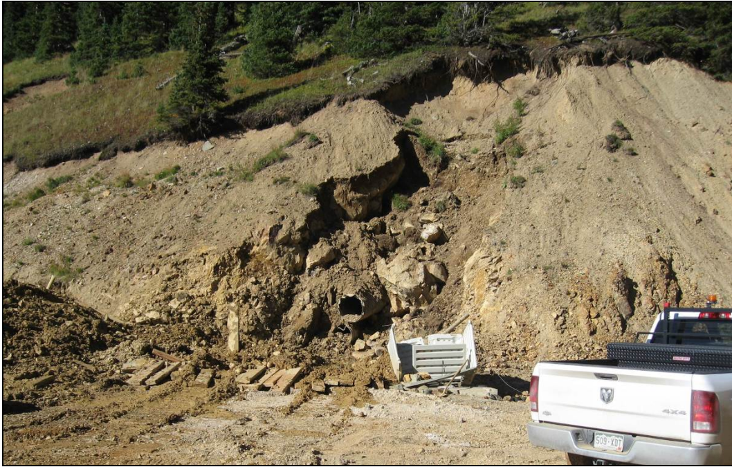
Figure 25.—Photograph showing excavation of the Gold King Mine New Adit portal on September 11, 2014. The metal grating and portions of the upper corrugated HDPE pipe and the lower solid-wall drain pipe have been removed (photograph from EPA project files).
