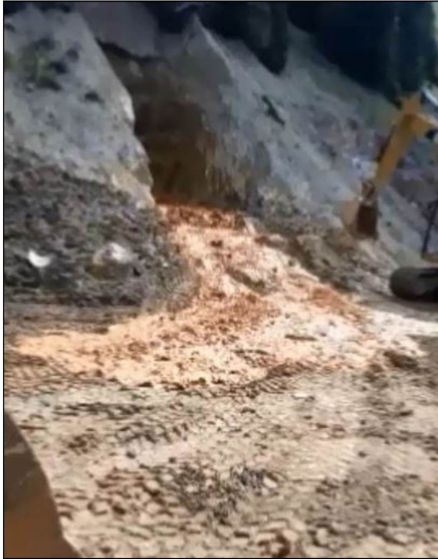
Figure 52.—Photograph showing the initial blowout from the adit. At this point, the flow is surging up over the backfill that was present in the portal area (still frame extracted from a video taken on August 5, 2015, at approximately 10:55 a.m.).
